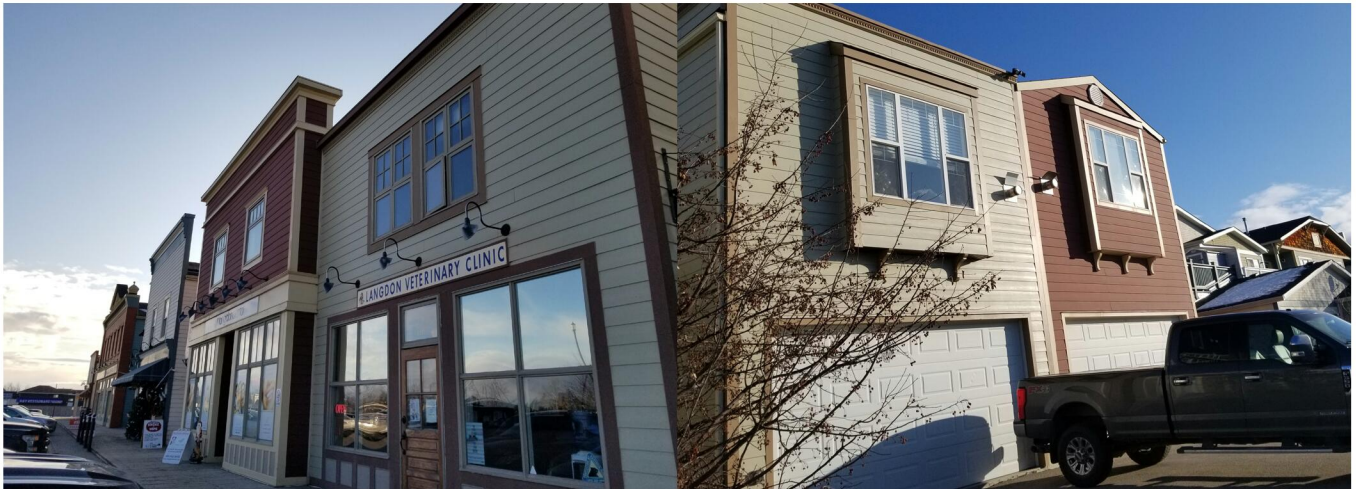
Figure 13: An example of a multi-use commercial and housing development (Langdon, Alberta – 2020)
